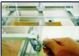
Place the two End brackets properly in position. Push the end brackets into the ceiling structure rails and check the end brackets sit securely on the rails.
